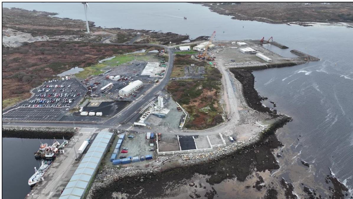
Figure 22: Photograph on the 14th Dec 2023 View of Compound, Concrete Batching Plant, Aggregate Storage Areas in foreground with works area in background.
