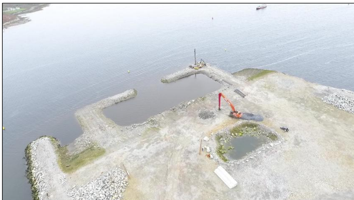
Figure 14: Progress with blasting platforms on 11 Oct 2023.
