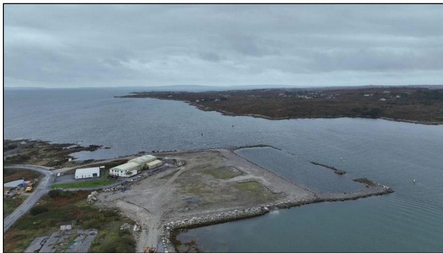
Figure 6: Status of site on 29th October 2024.
