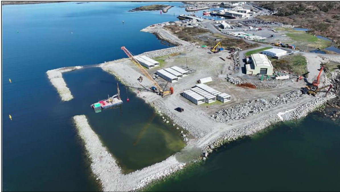
Figure 15: Quay wall trench and protective berm on 20th March 2024.
