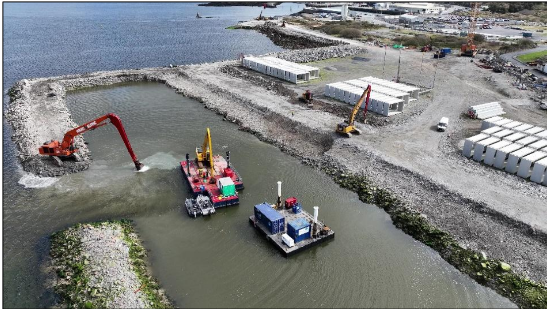
Figure 17: Photograph showing use of excavators on the protective berm and on floating pontoons in the constructed lagoon.
