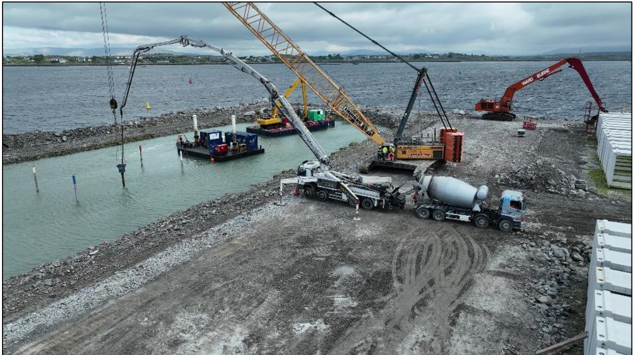
Figure 20: Liquid concrete being delivered via Tremie Pipe and directed by underwater divers to surround and hold the foundation beams in place.
