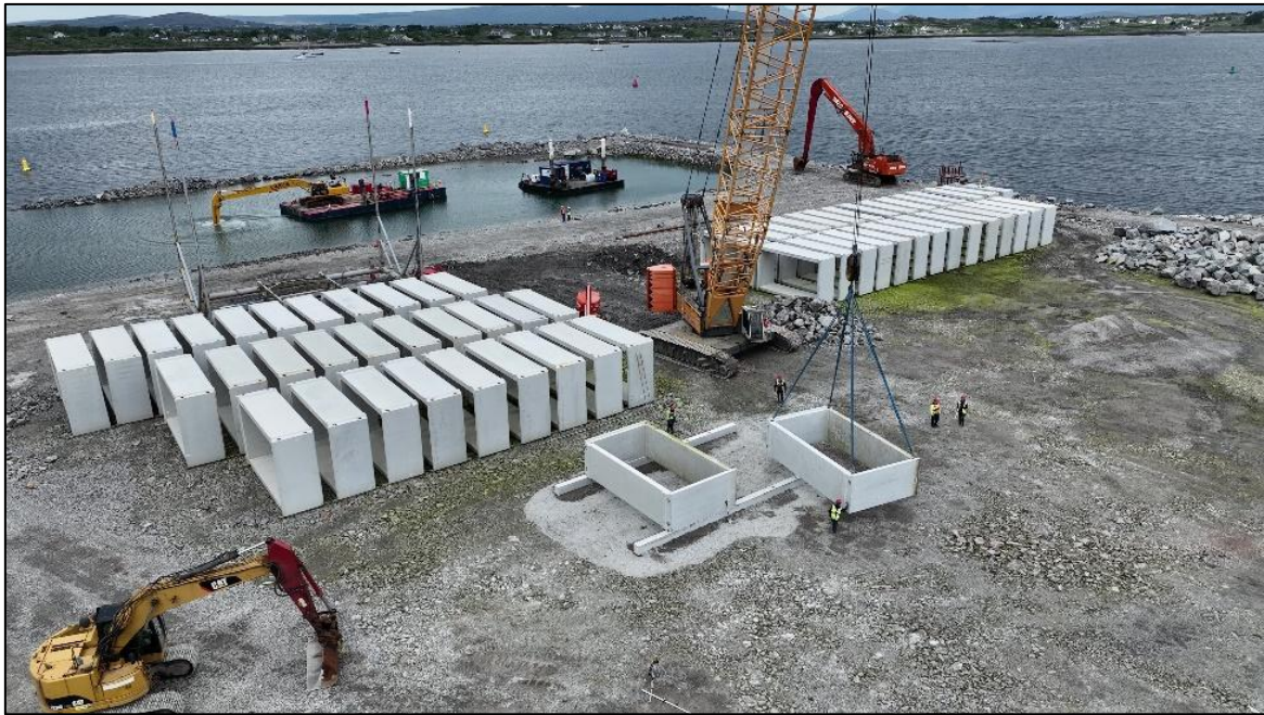
Figure 18: Photograph showing the (7m x 4m x 2m) concrete caisson boxes being positioned on precast concrete foundation beams positioned on the ground during a field trial on land.
