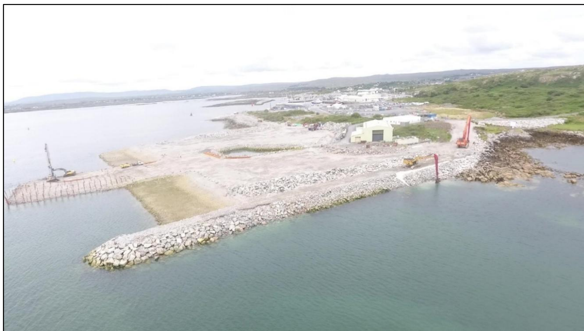
Figure 11: Southern protective berm with initial 3 blasting platforms in the middle of the quay wall trench on 12 July 2023.
