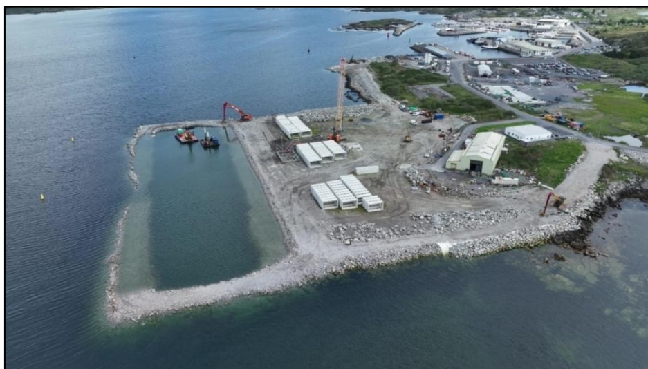
Figure 8: Site Status on 14 May 2024 when the presumed lawful works ceased.
