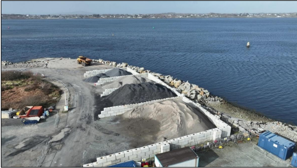
Figure 25: Storage areas for the construction materials and supplies for the concrete production plant adjacent to the construction compound.
