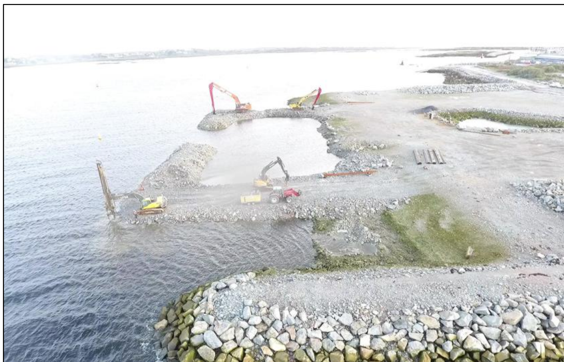
Figure 13: Construction of two blasting platforms on 26th Sept 2023.
