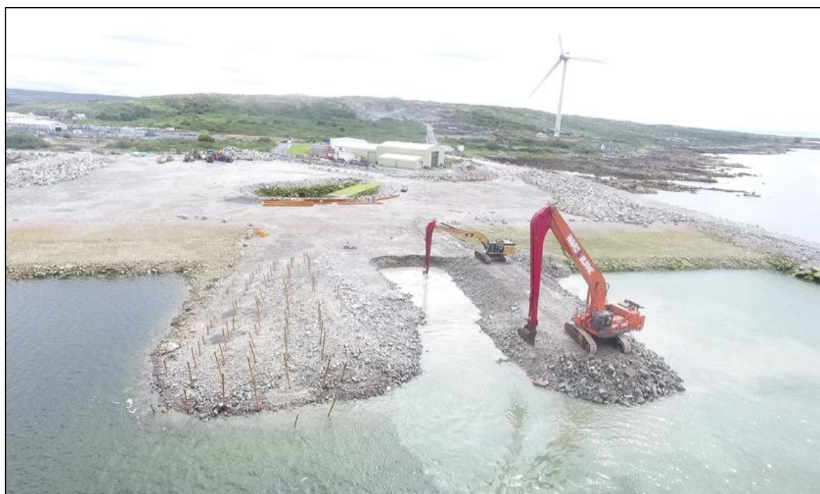
Figure 12: Construction of blasting platform 5 on 18th July 2023.
