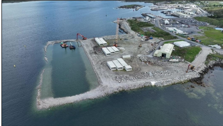
Figure 5: Site Status on 20 th May 2024 when the works ceased.
