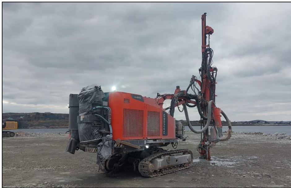
Figure 16: Drilling Rig used to drill the blasting holes.
