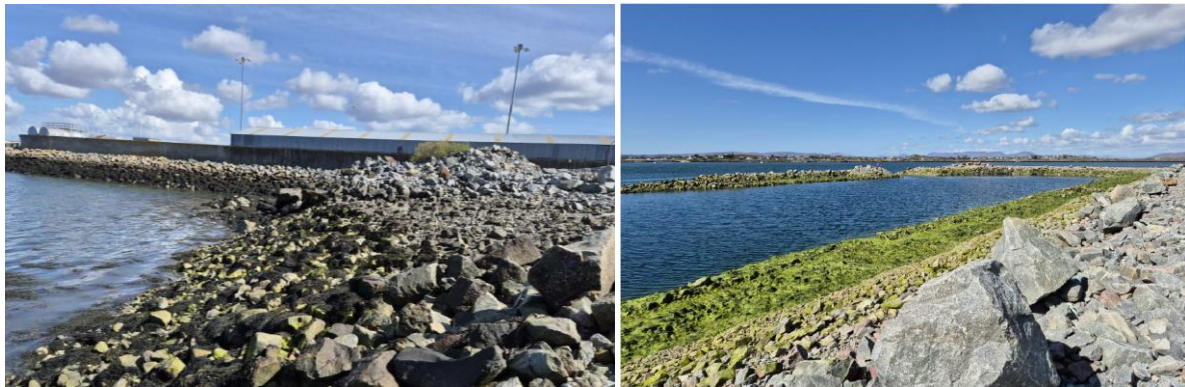
Plate 2. Sea Walls, Piers and Jetties (CC1) and Open Marine Water (MW1) – (left) at northeast corner with Pier 1 in background, and (right) rectangular rock berm with green seaweed ( Enteromorpha spp.) layer.
