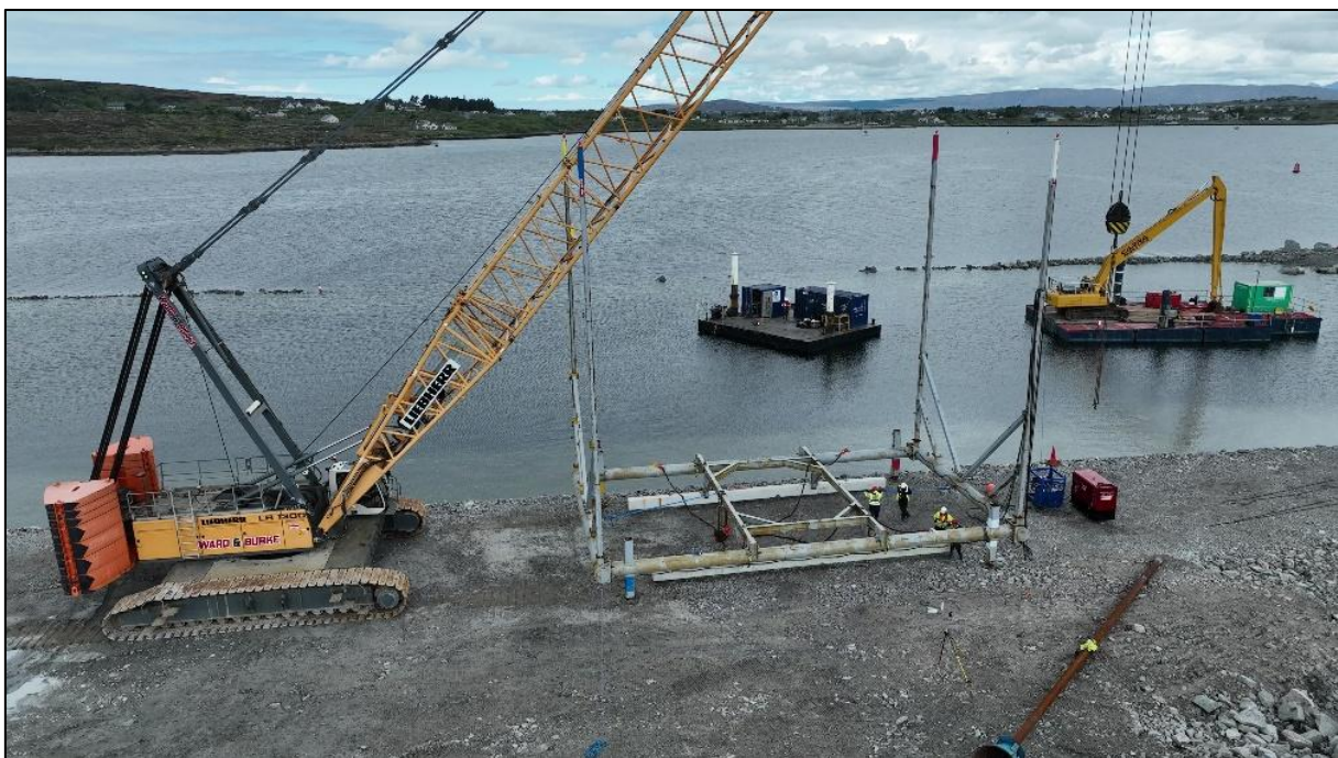
Figure 19: Bespoke frame used to accurately lower and position the foundation beams for the quay wall in the trench.
